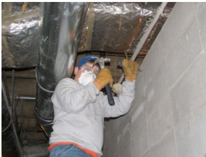
It was hard to get started because the walls were built well and we didn't use any power tools, for safety reasons.
